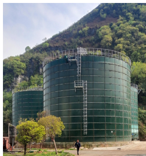
3 sets of 5000m 3 CSTR Tanks for Agricultural Waste
