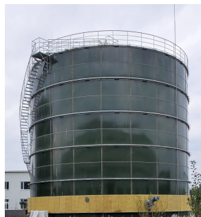
1800m 3 UASB Tank for Wastewater from Hebei Pharmaceutical Factory
