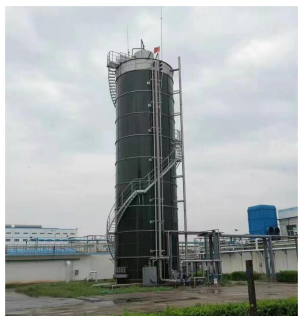
Xinjiang Enterprise Sewage Treatment 1500m 3 IC Tower
